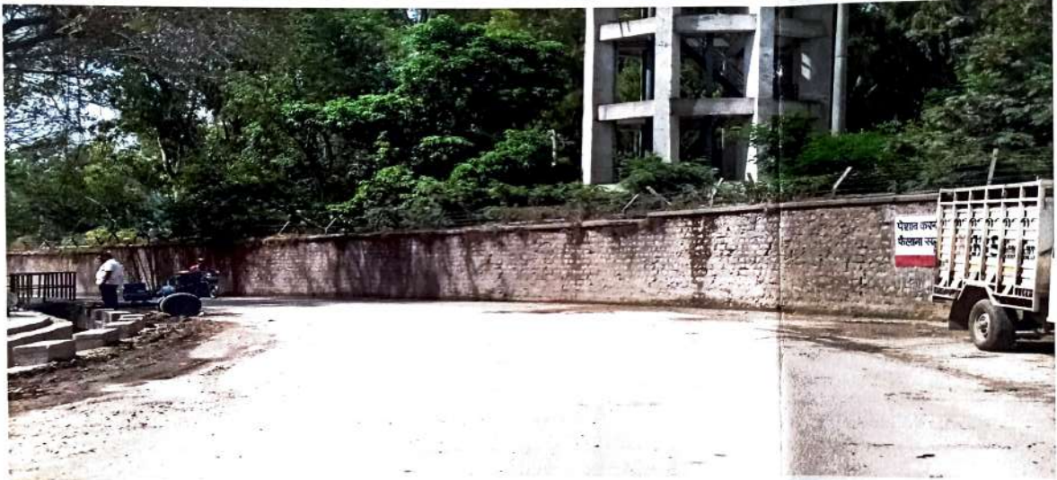
Picture of Road after Cleaning
