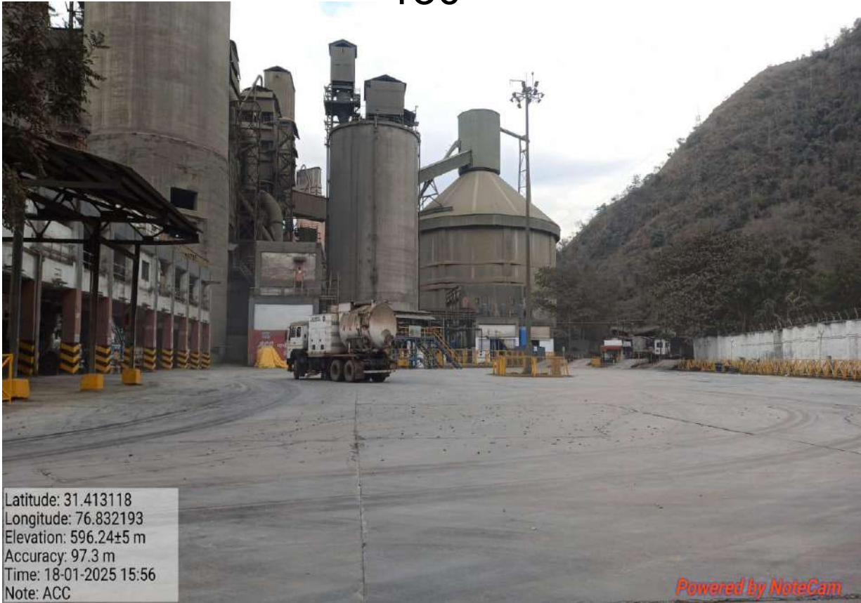
Cement Silos, Fly Ash Silo, Clinker Silo (Left to Right)
