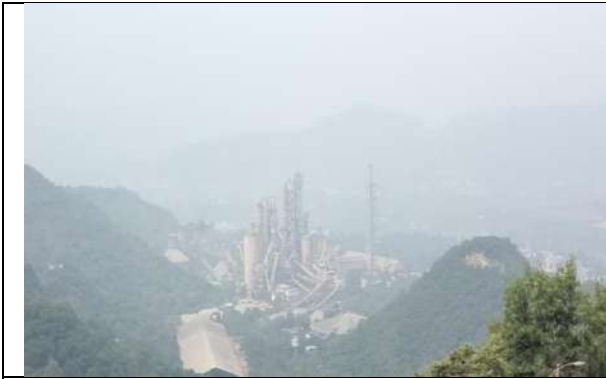
Photo 1- A view of cement plant from mining area
