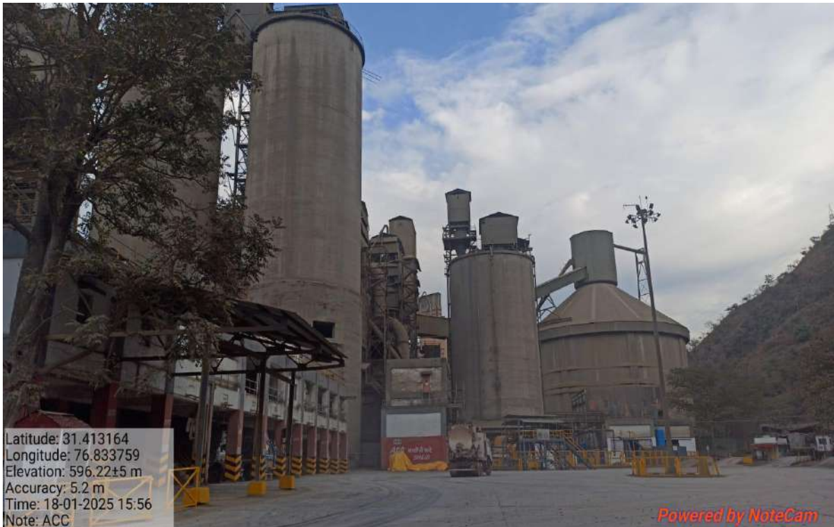
Cement Silos, Fly Ash Silo, Clinker Silo (Left to Right)
